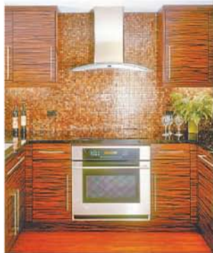
Low-emission dark quartz countertops were selected for use in the kitchen, as were more recycled glass mosaic tiles.
