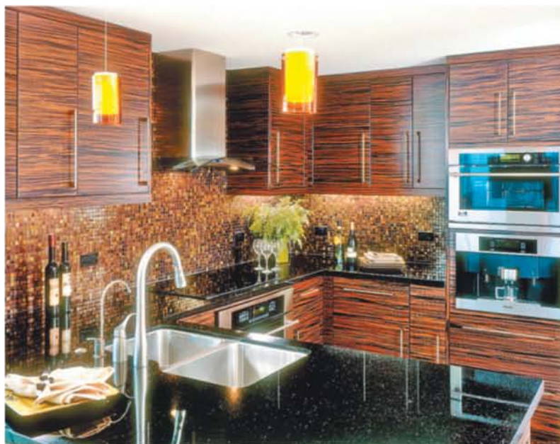
Cabinets in the kitchen are made of a composite veneer to give them the streaked look of Macassar ebony, a rare hardwood from Indonesia. The dishwasher and faucets were selected for their water efficiency and the refrigerator for its low energy use.
